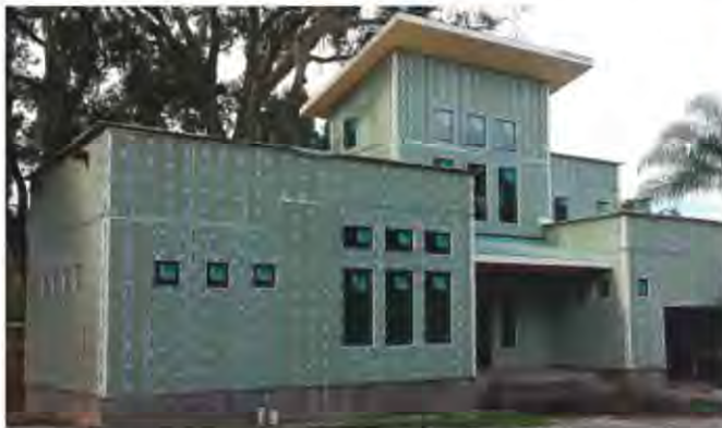
HercuWalls for a 2,400-sq.-ft. production house can be installed in 2.5 hours and concrete placed in two more hours with a crew of five.
