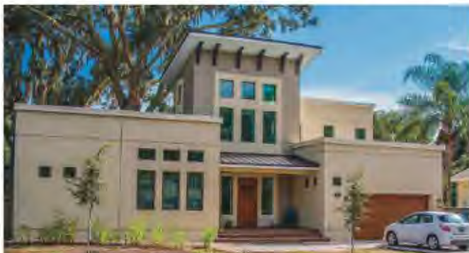
HercuWalls for a 2,400-sq.-ft. production house can be installed in 2.5 hours and concrete placed in two more hours with a crew of five.
