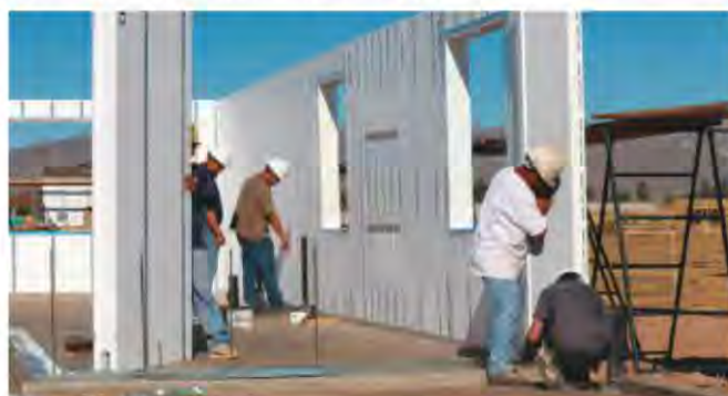
HercuWall is delivered to the jobsite as a kit of ready-to-install panels, eliminating the necessity for any job-site modification.
