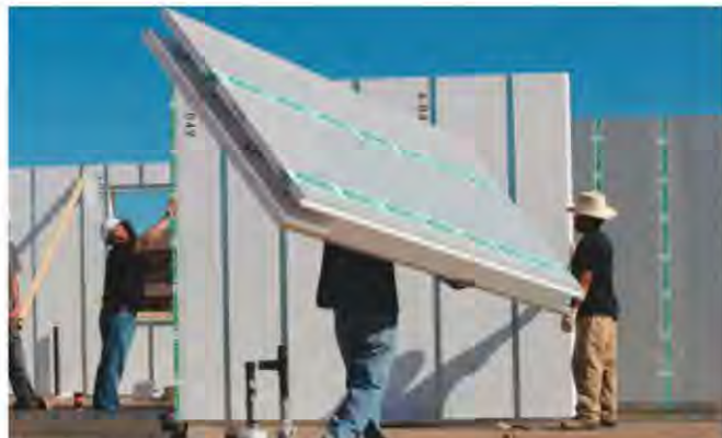
HercuWall is delivered to the jobsite as a kit of ready-to-install panels, eliminating the necessity for any job-site modification.
