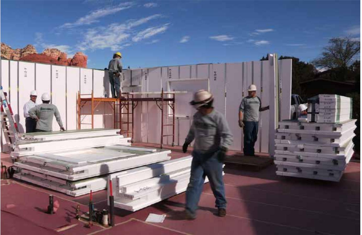
The HercuWall panelized wall system was installed in Sedona without costly special equipment. Photo courtesy HercuTech.
